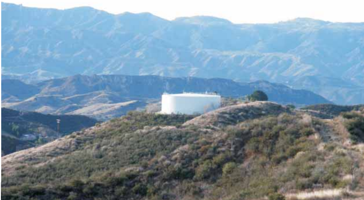
Photograph of water tank looking east from southeast part of project site.
