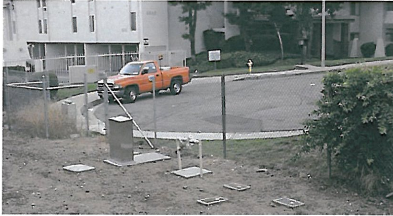
Clustering roadside facilities at safe locations away from traffic minimizes worker exposure to traffic.
